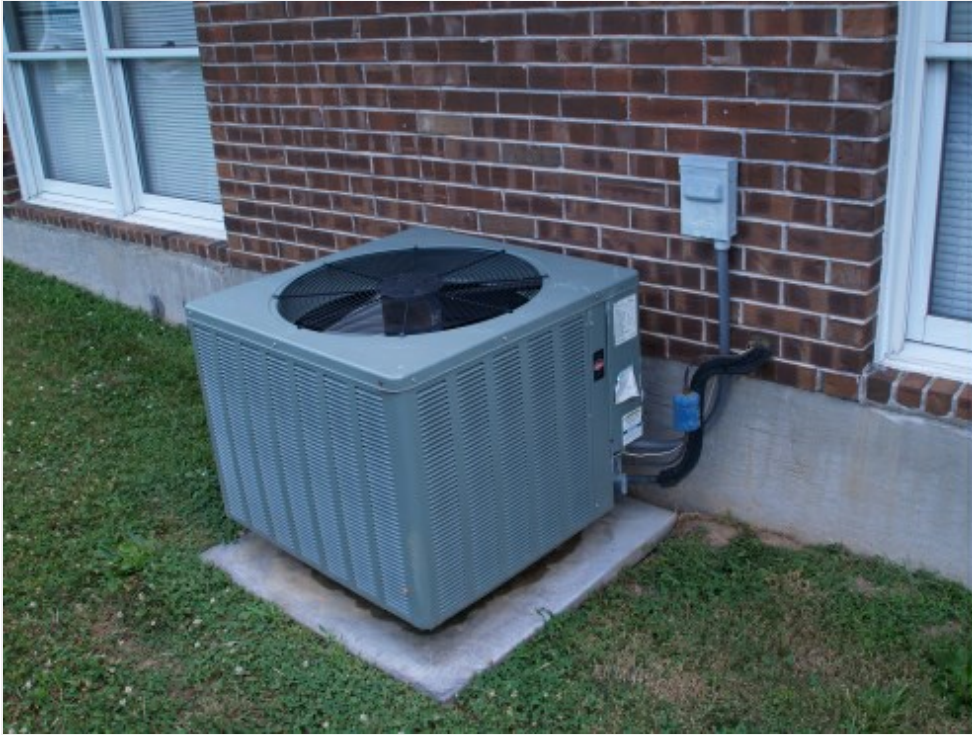
One of the AC condensers
